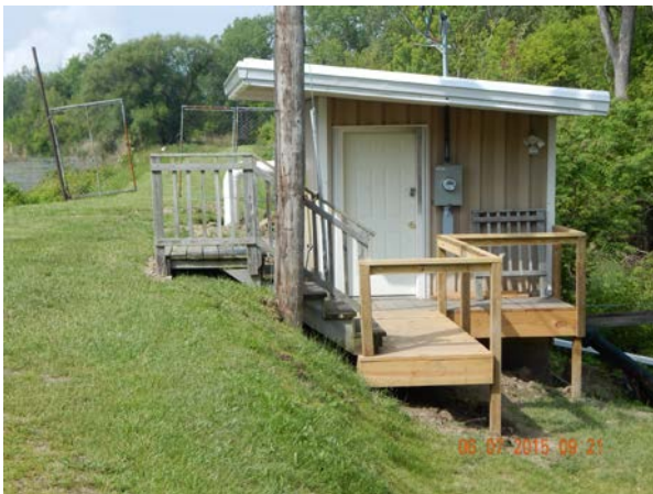
Pump House Looking South along Dike
