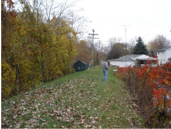
Dike Picture Looking North
