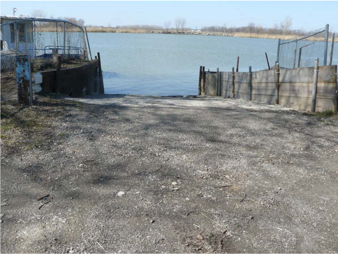
Looking West Down Boat Ramp
