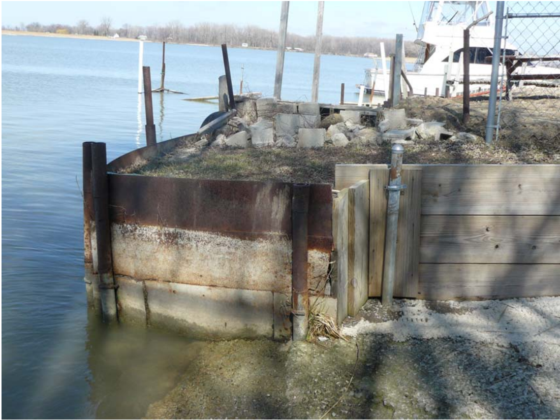
Looking at Northwest Corner of Boat Ramp
