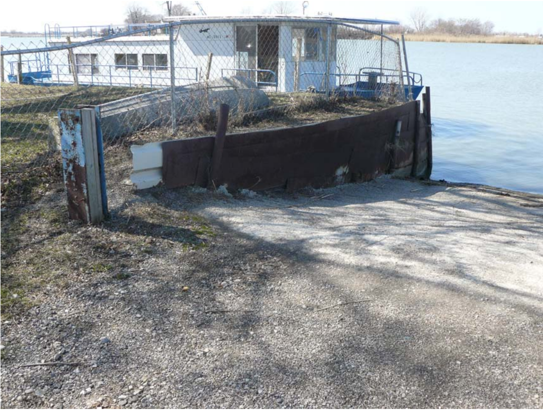
South Wall of Boat Ramp
