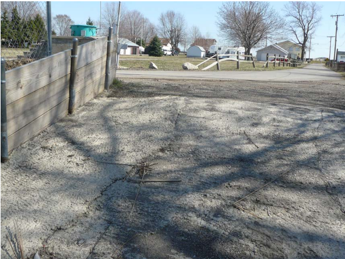
Looking Up Boat Ramp at Lakeshore Drive
